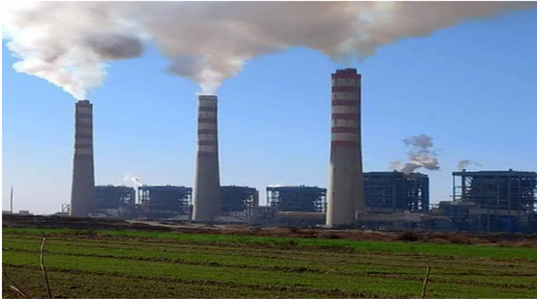
Figure 1. The Wassit thermal station.
